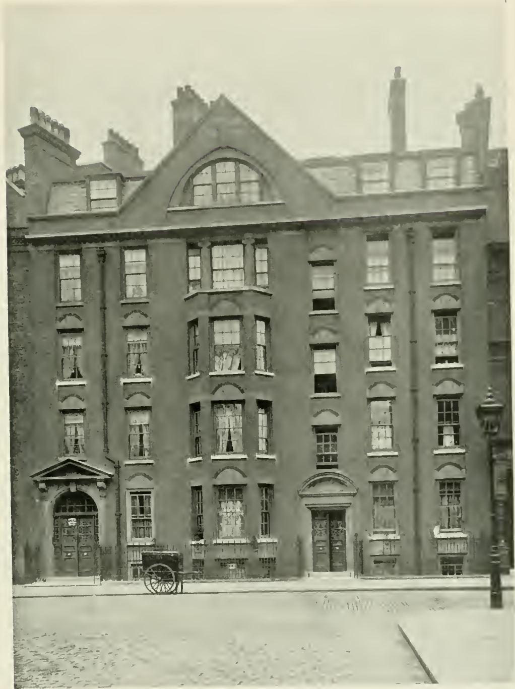
NOS. 18, 19, AND 20, FOLEY STREET, LONDON, W. AN EXAMPLE OF INEXPENSIVE STREET FLATS HAVING THE CHARACTER OF GOOD TOWN HOUSES IN A NEIGHBOURHOOD WHERE HIGH RENTS ARE NOT TO BE OBTAINED. THE MATERIALS ARE RED BRICK AND PORTLAND STONE. A PLAN OF THE GROUND FLOOR IS GIVEN ON PAGE 42
